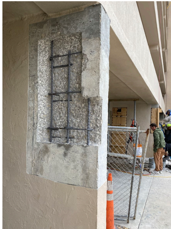
Picture 2: Typical divider wall repair
