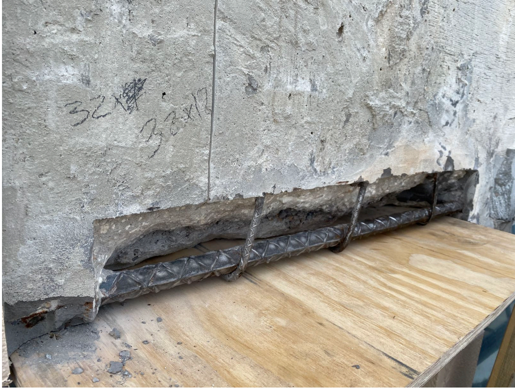
Picture 1: Unit 605 header repair
