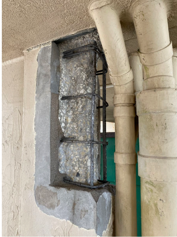
Picture 3: Typical divider wall repair
